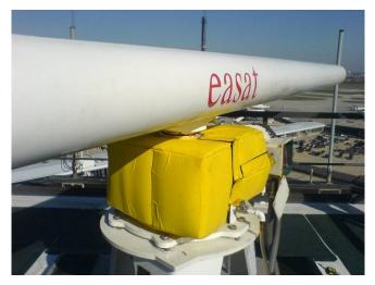
Therm<sup>™</sup> liner. The project was a success. No more vibrational noise!!! In fact the highly efficient insulation cover was able to retain nearly all of the internal heat generated inside the gear box so that the conduction heating pad was rarely required.
